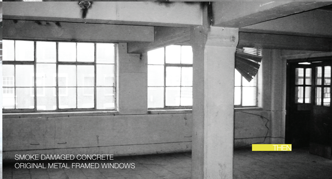
TYPICAL FLOOR: EXPOSED BACON FAT RIDDEN COLUMNS AND FLOOR. CLEAR AREAS INDICATE WHERE ORIGINAL BLOCKWORK PARTITIONS STOOD.
