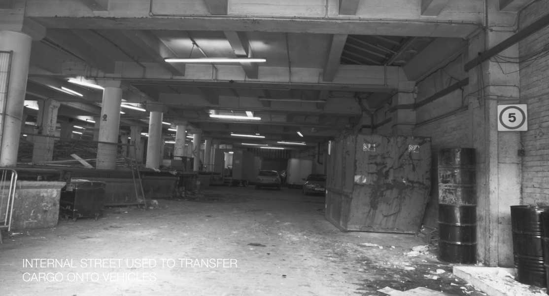
TYPICAL FLOOR: EXPOSED BACON FAT RIDDEN COLUMNS AND FLOOR. CLEAR AREAS INDICATE WHERE ORIGINAL BLOCKWORK PARTITIONS STOOD.
